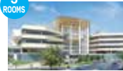
UNIVERSITY OF PENNSYLVANIA HEALTH SYSTEM ROBERTS PROTON THERAPY CENTER Philadelphia, PA, USA Treating since 2010
