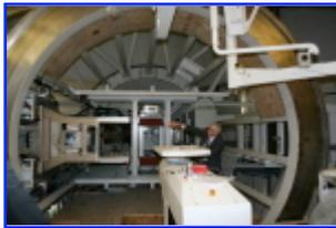
**A treatment room under construction reveals the beam entry site into the gantry area**
